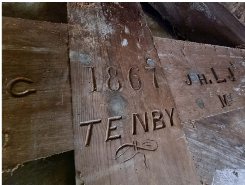
A message from our Victorian predecessors, hidden high in the gloom of the roof trusses
