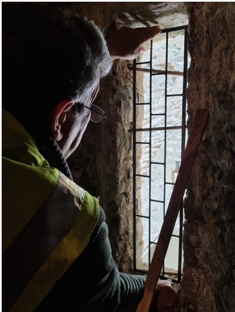
Glazier Bruce Brockweir installing new windows
