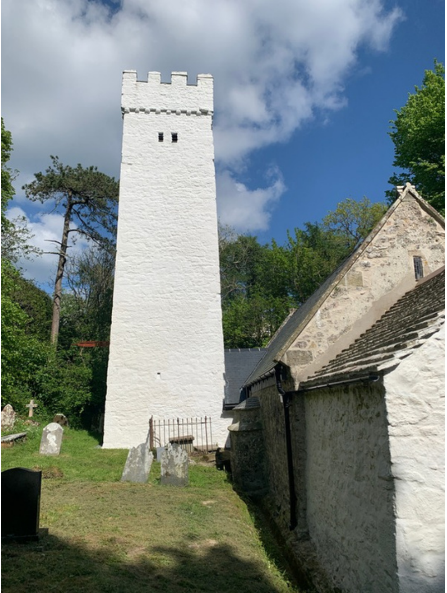
The church tower in its gleaming coat
