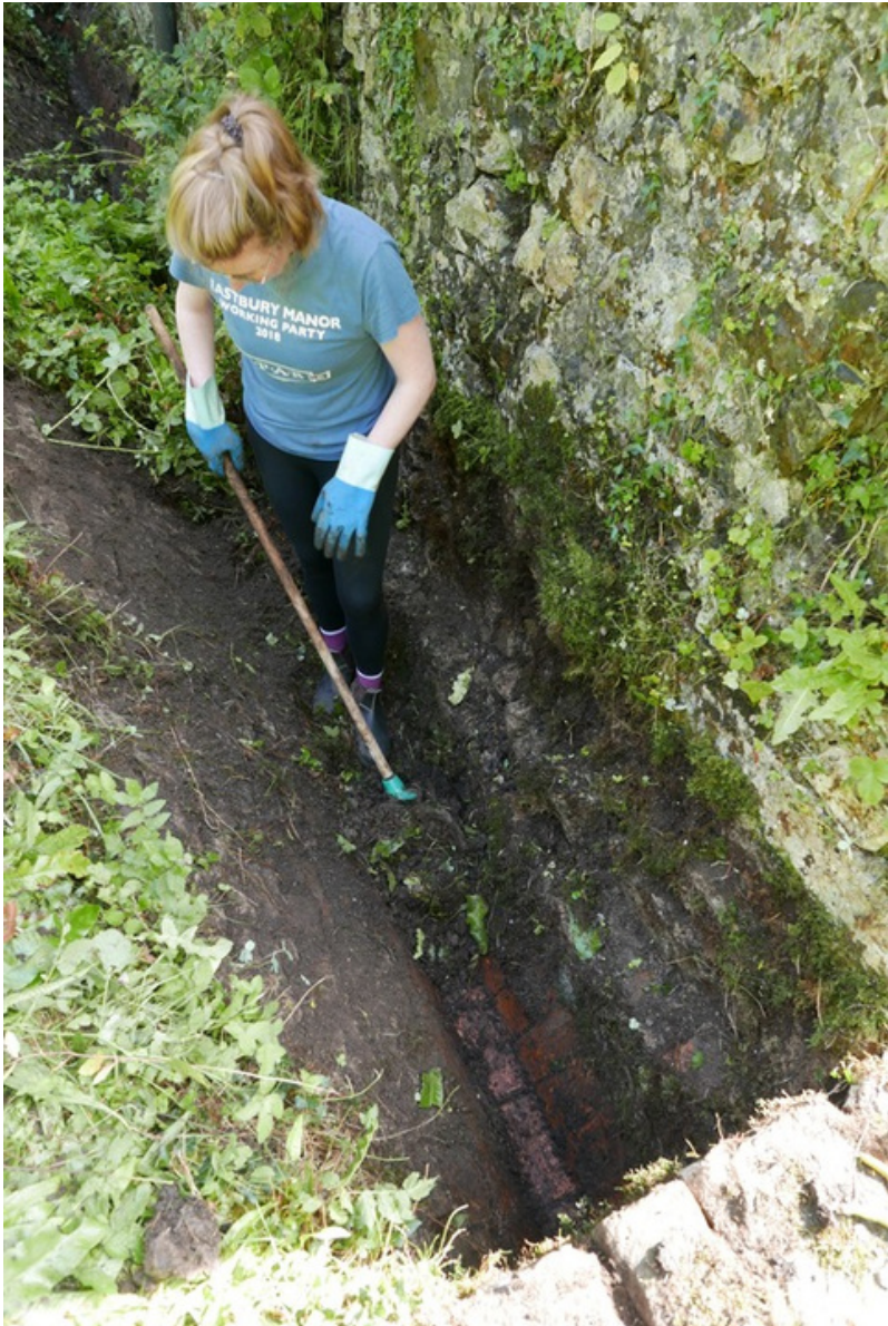
Rachel digging out the north drainage channel
