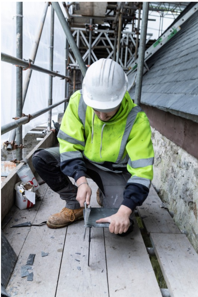
Dressing slates ready for the new roof
