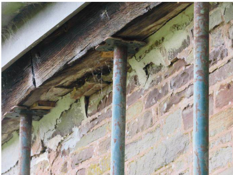
Top: Scaffold poles supporting the wall-plate on the north side Bottom: Showing extent wall-plate had pushed off the stone wall
