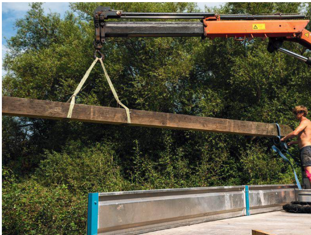
A new oak wall-plate is delivered to site
