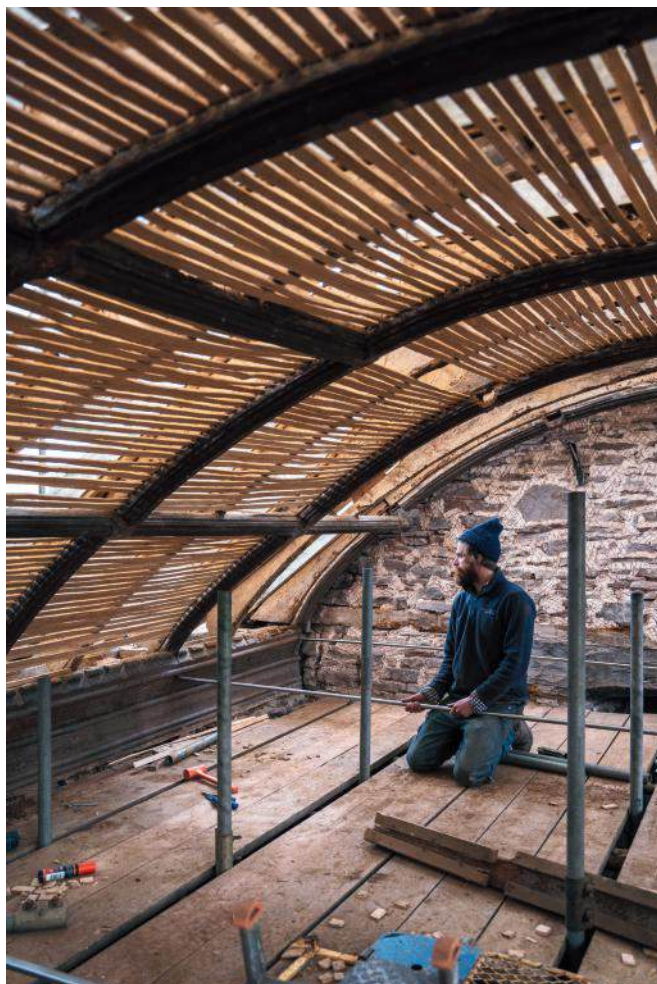
The roof is back in alignment and the laths have all been inserted, ready to be plastered. Jack adjusting a new stainless steel tie-bar.
