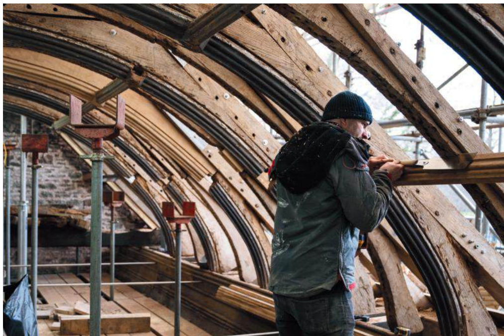
Joe carefully adjusting a newly carved rib
