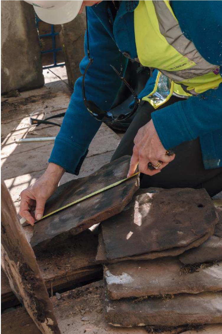
Measuring and organising tiles to create a slope of tiles gradually diminishing in size
