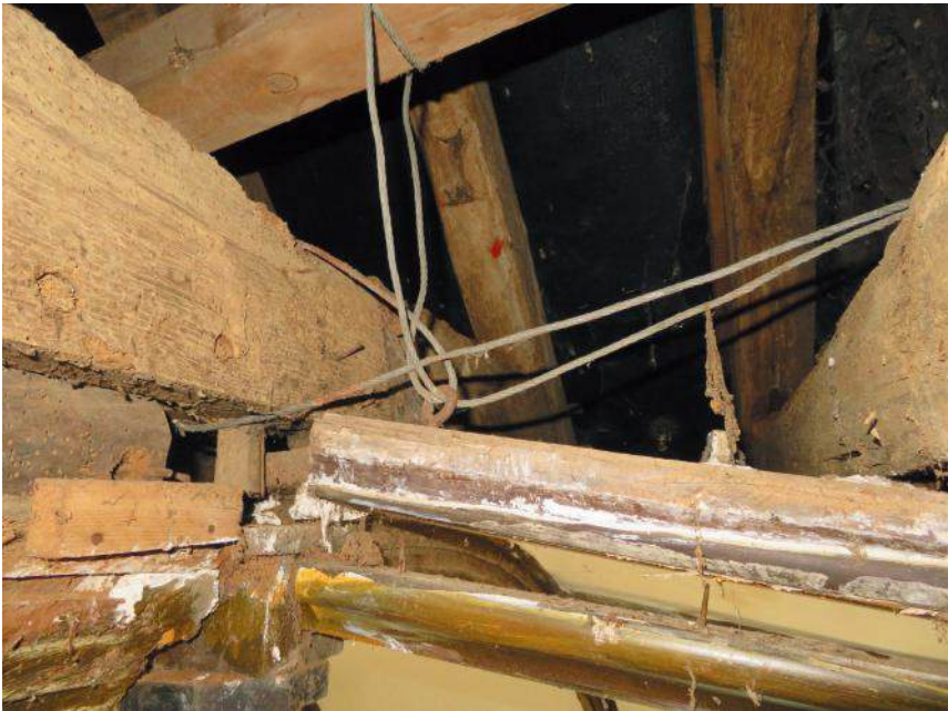
Snapped trusses
