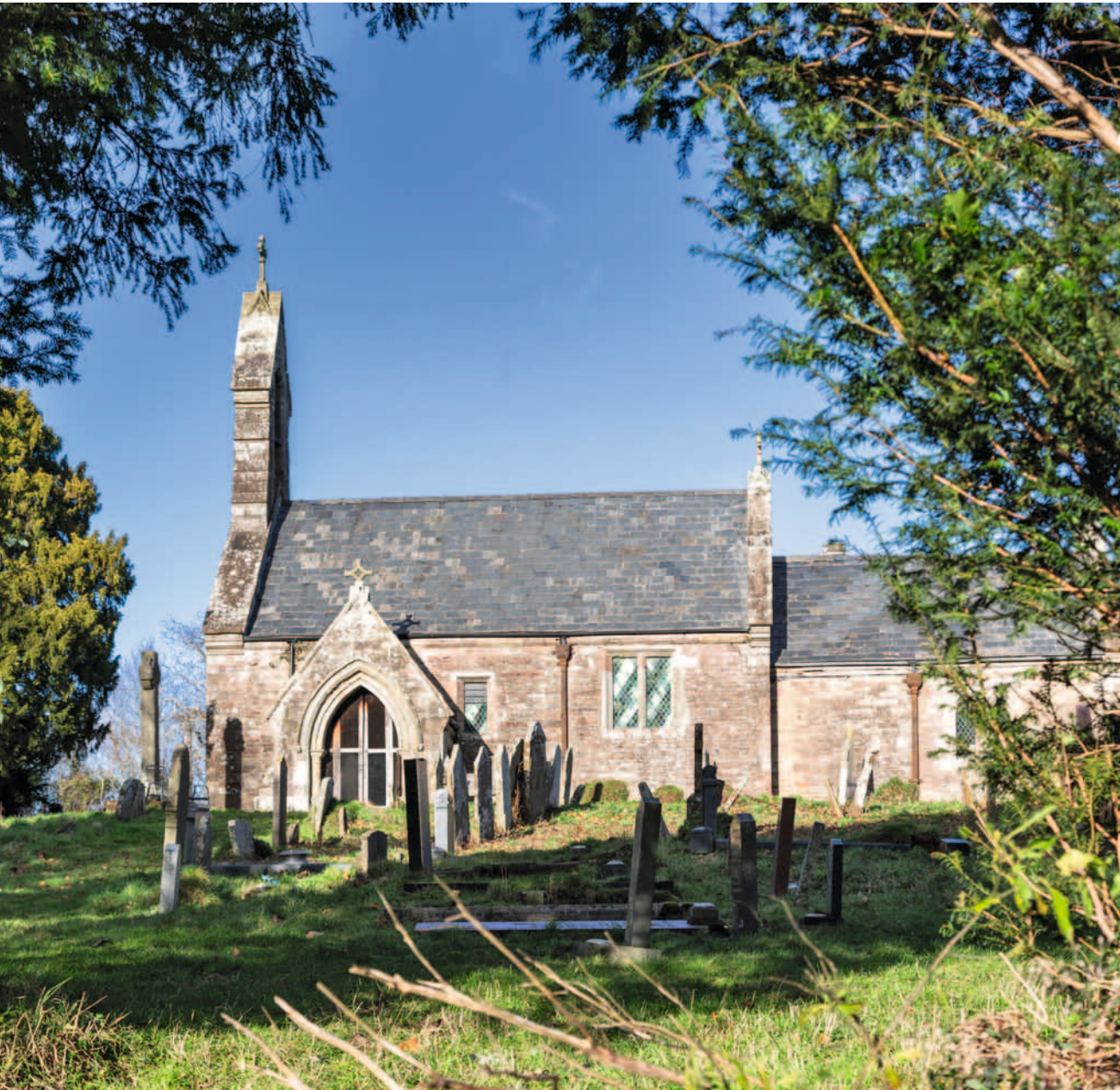
South elevation of St Mary's, Kenderchurch.
